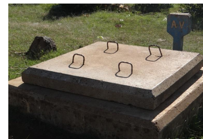
Plate 2: A sewer line within Elgon View estate
