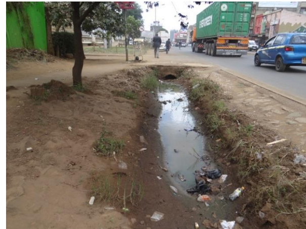
Plate 5: No provision of storm drains on the road
