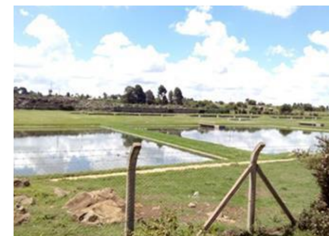
Plate 1: The sewer plant at Kipkenyo
